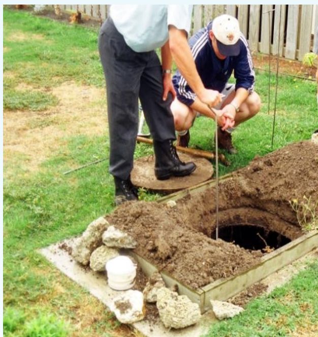
Checking scum and sludge levels in a septic tank
